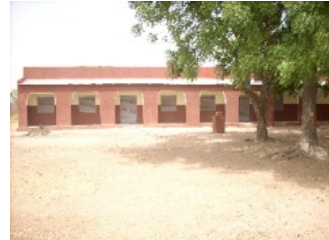
New Middle School, Diaka, completed Feb. 2009
