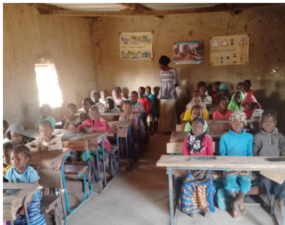
The old schoolrooms in Koro N'Tossoni, in a mud brick building built by the community
